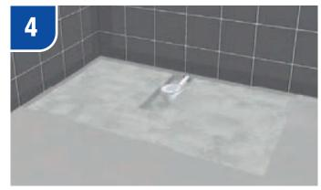
Remove DEC. It will be necessary to remove an area to sufficient depth under the outlet position to accommodate the shower trap.
