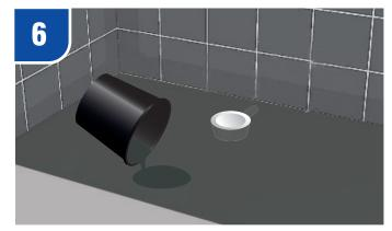
Apply a 'weak' sand and cement mix to the proposed area. This will ensure DEC is fully supported.
